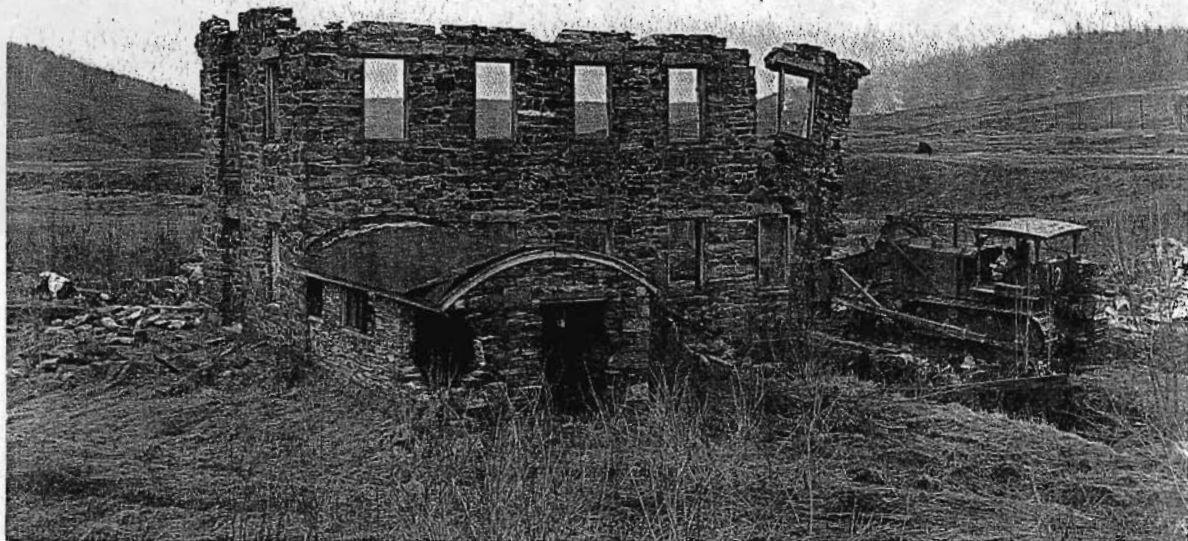
Pushing down the Old Stone Mill, Enfield
