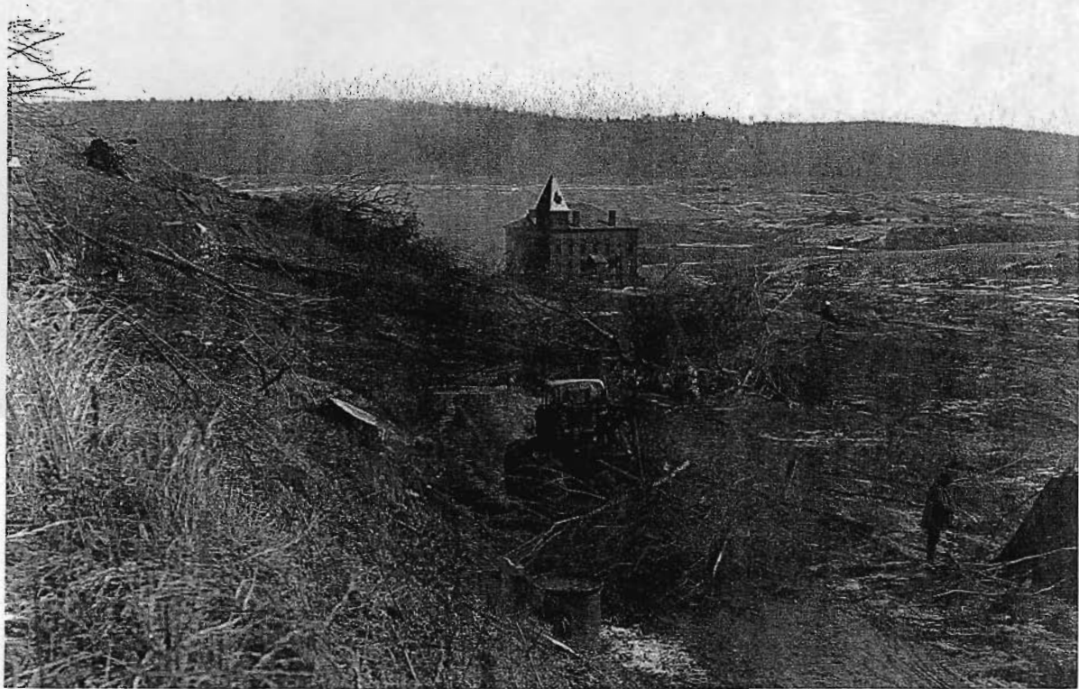
Enfield, February 1939. The town hall still stands; the town is gone.
